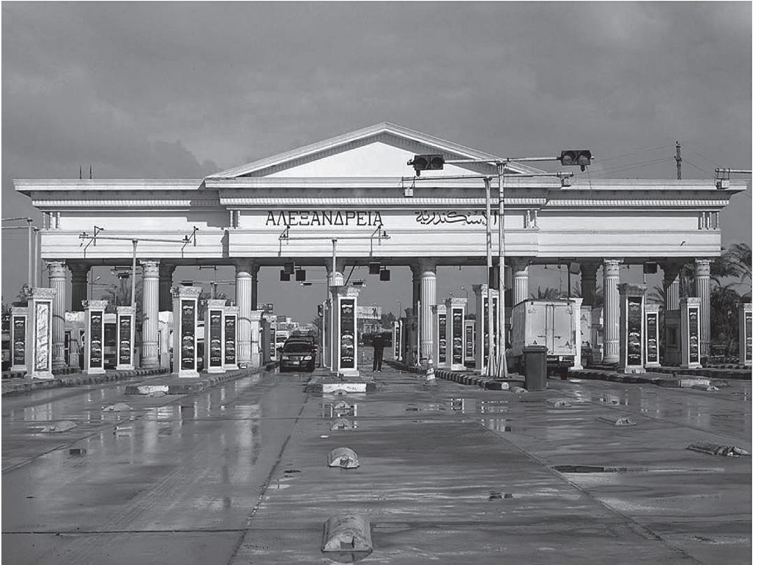
The neoclassical toll booths on the Desert Road leading in and out of Alexandria Governorate.
